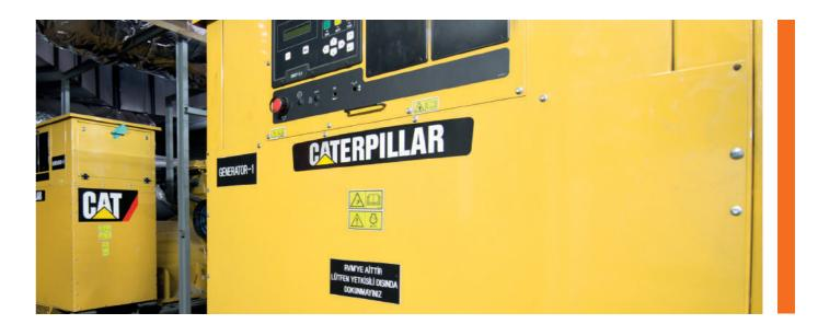
The Synchronization Control Grid follows the power flow instantly for the transitions (generator-generator, transformer-transformer and generator-transformer) and conducts the transitions automatically in cases of breakdown, low/insufficient voltage or frequency. The UPS infrastructure steps in during transitions, which can last up to 30 seconds, providing uninterrupted power supply. The battery pack of the UPS system has a minimum runtime of 15 minutes.
